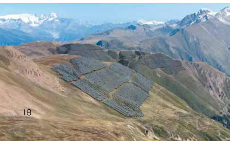
GrengiolsSolar - a pioneering project for high-alpine photovoltaics in the Saflisch valley of Upper Valais.
